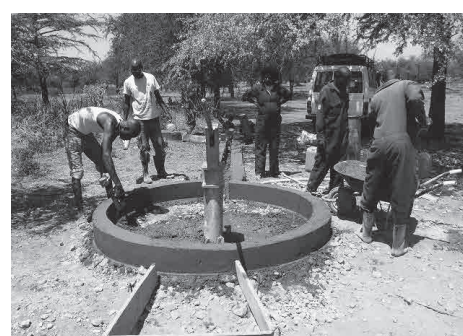
With the support from AAR Japan, residents work with water well-maintenance technicians to repair water wells in the area. (October 2015)
