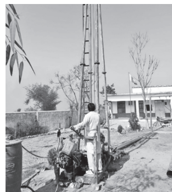
Drilling a well at a girls' elementary school in a mountainous area to secure a water source for toilets and hand-washing (February 2022)
